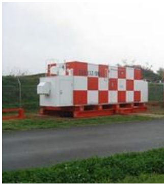
Figure 2.6.2 [Installation of equipment]
